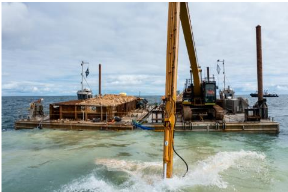
Figure 32: Deploying rocky reef base in Port Phillip Bay, Victoria, November 2021 (Photo credit: Streamline Media).
