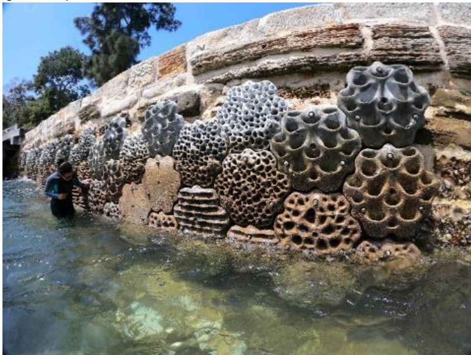
Figure 41: Series of engineered panels attached to seawall increasing habitat complexity. Photo: Alex Goad
