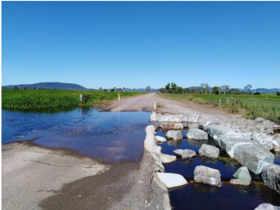
Figure 43: Engineered fish ladder designed to reconnect floodplains for successful fish passage
