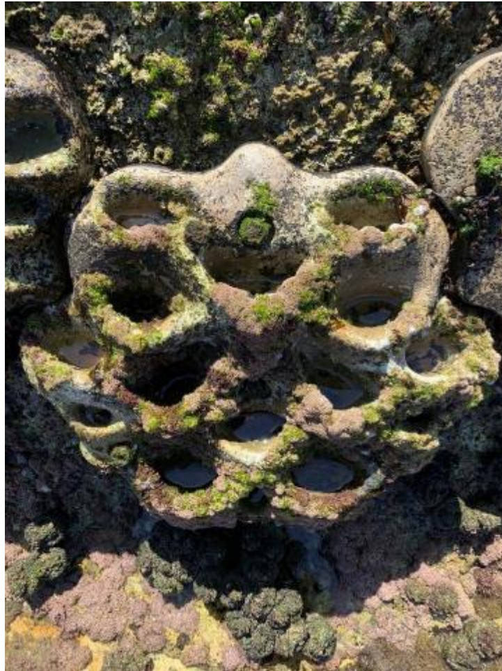
Figure 40: Engineered panel for seawall. Photo: Maria Vozzo
